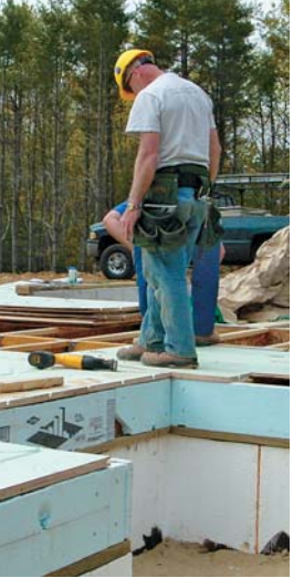
ABOVE: Insulated concrete forms were used for the home's foundation.
