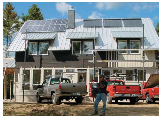
ABOVE and RIGHT: Cranberry Ridge features solar electric and solar water-heating systems on its roof.
